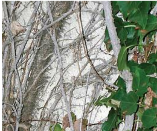
Fig.1 Boundary Ivy attaches to a building using aggressive adhesive suckers or climbing roots that can damage surfaces and enter voids and cracks
